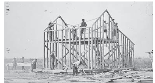
The Parsonage likely has balloon framed construction because it was built in the 1870s. This image shows the studs running from the foundation to the roofline. IMAGE: Omaha Reservation, Nebraska, 1877 © William Henry Jackson; The National Anthropological Archives, Smithsonian Institution
